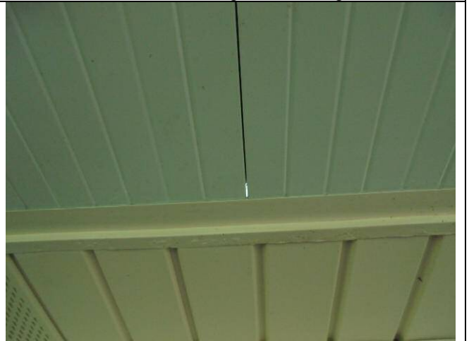
A proper flashing should be provided at the intersection of the exterior wall of the house and the deck/porch cover.
